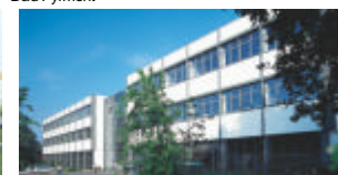
PHOENIX CONTACT ELECTRONICS Bad Pyrmont
